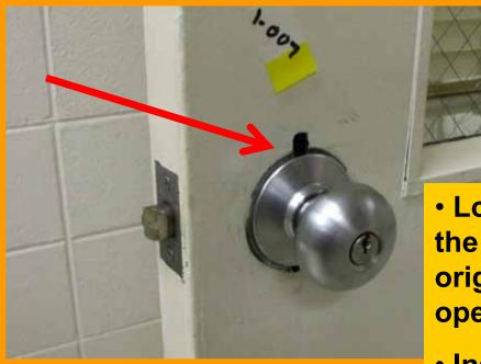
• Lock has been changed, and the new lock does not cover the original holes on this fire rated opening.
