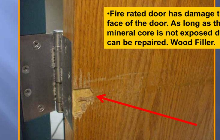
•Fire rated door has damage to the face of the door. As long as the mineral core is not exposed door
