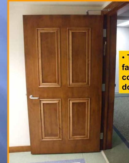
• The molding (plant-ons) were factory applied, which does conform with NFPA-80. This door is OK.
