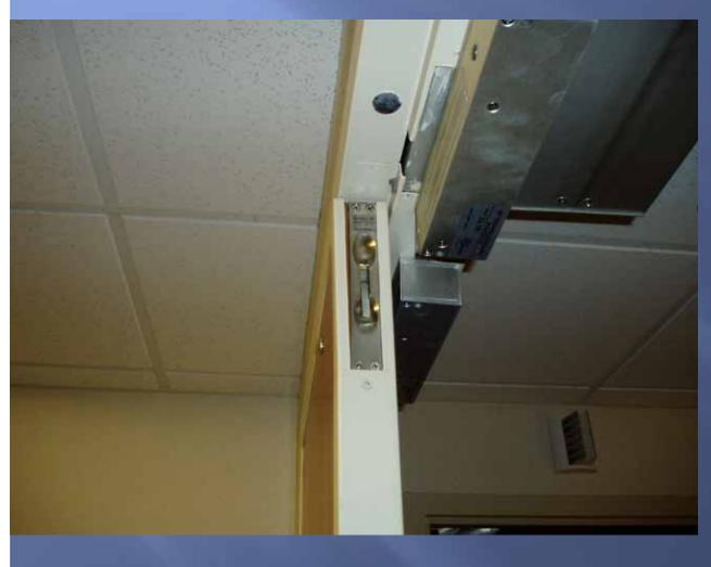
Fire Doors require Automatic Flush bolts. Magnetic Locks with no Positive Latching hardware.
