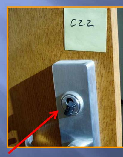
• Fire rated door, the lock is missing its cylinder and should be adjusted to its proper function.
