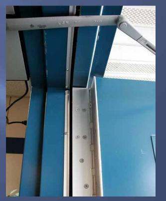
On doors with a continuous hinge, the fire label should be on top of the door and frame header.
