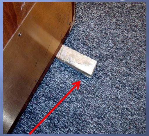
Wedge under door prevents door from closing in a fire or <u>emergency situation</u>.
