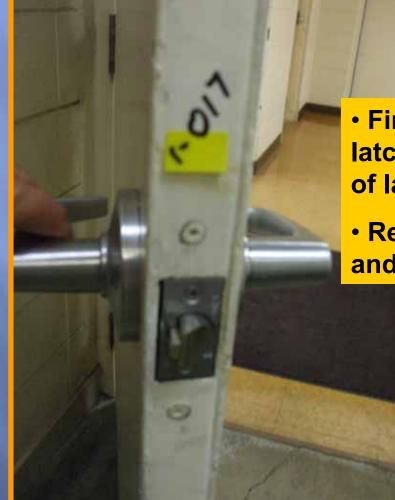
Fire rated door has a loose latchbolt and screws on face plate of latchbolt.
