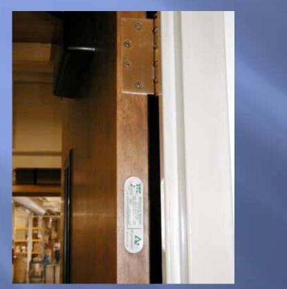
On doors with mortise hinges, the fire label should be approximately 6" below the top hinge.
