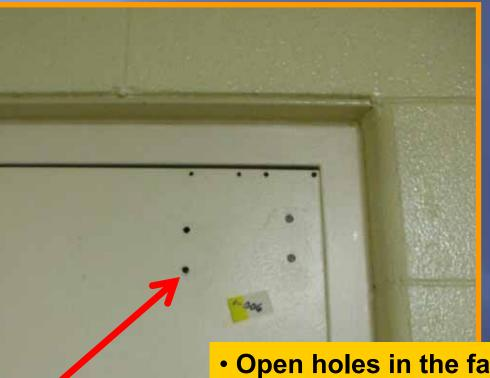
Open holes in the face of a fire rated door.
