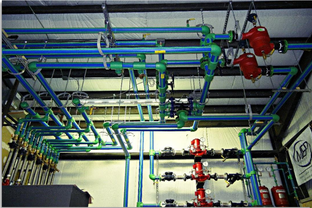
Geothermal Heating & Cooling
