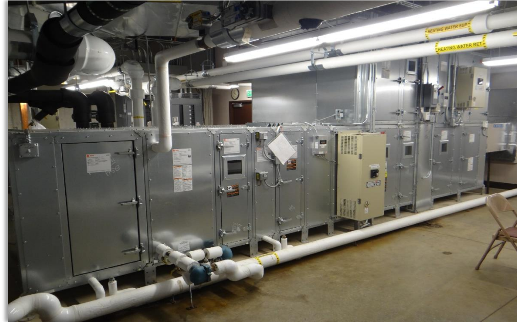
Energy recovery unit serving the demand based ventilation
