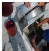
Sealing perimeter of ducting at RTE
