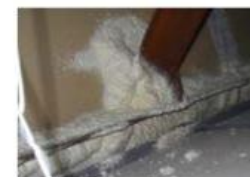
Air sealing above drop ceiling now provides a proper air barrier resulting in eliminating dirt entering the building at this detail, and increased occupant comfort.
