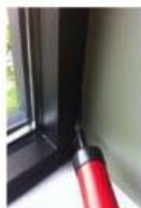
Testing window shows air infiltration before caulk.
