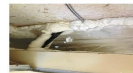
Soffit is blocked with insulated board and sealed with polyurethane foam.
