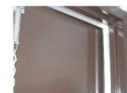
Exterior door has new quality weather-stripping.
