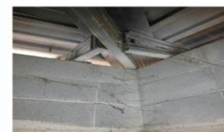
Large openings at soffit caused considerable energy loss and comfort-related issues. This was typical in most of the buildings.
