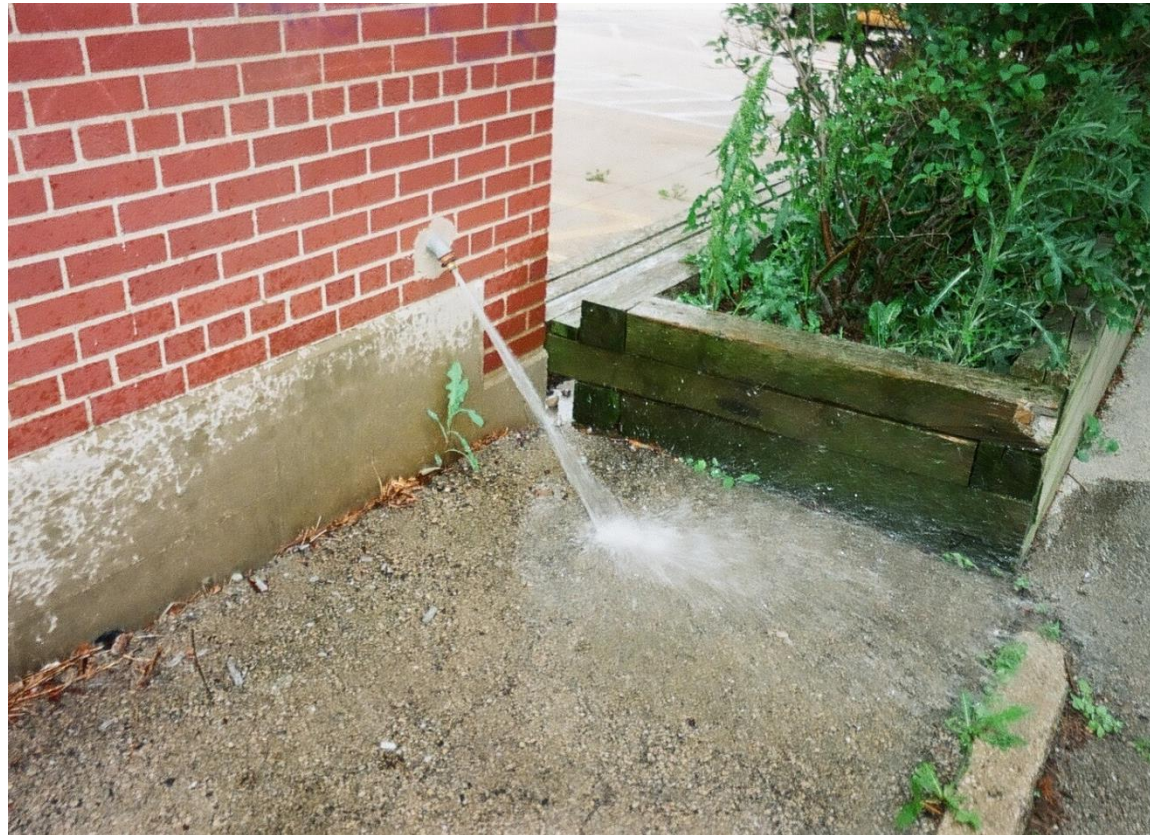
Inspector's Test Connection
