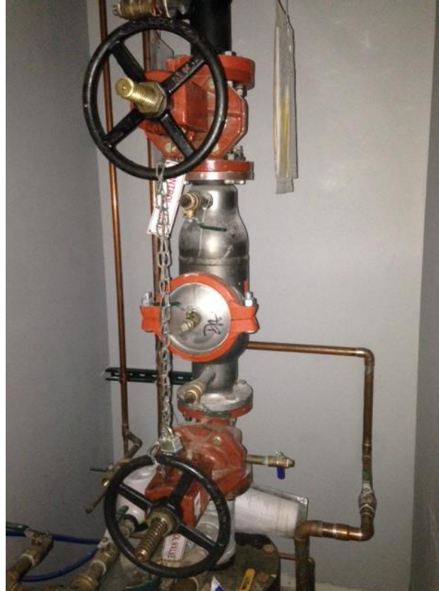
DC Backflow Assembly
