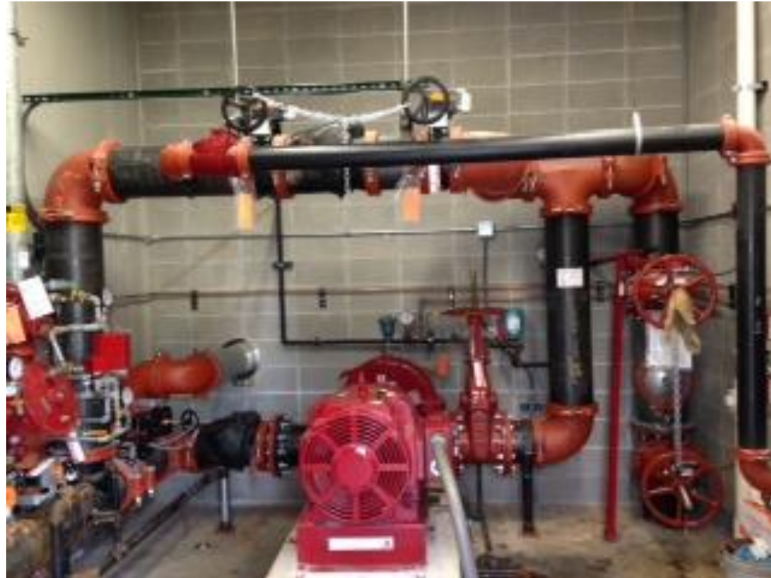
Electric Pump with Bypass
