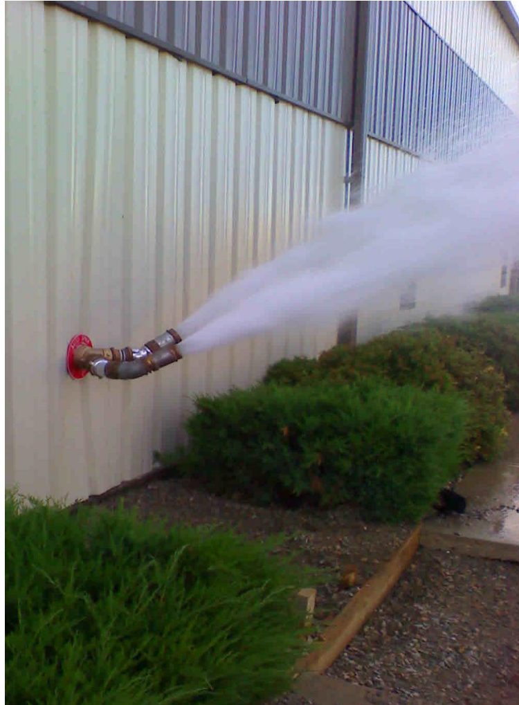
BFP Forward Flow Through FDC
