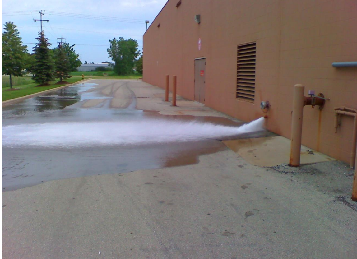
Main Drain Test Flowing
