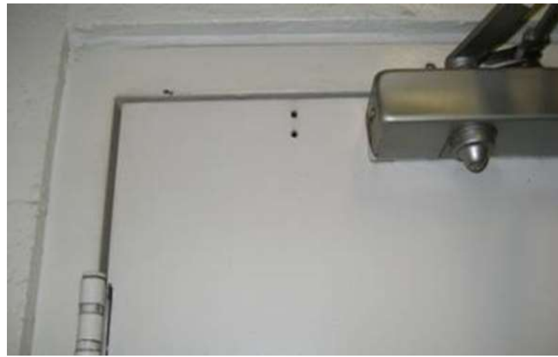
relocated closer exposing original mounting holes
