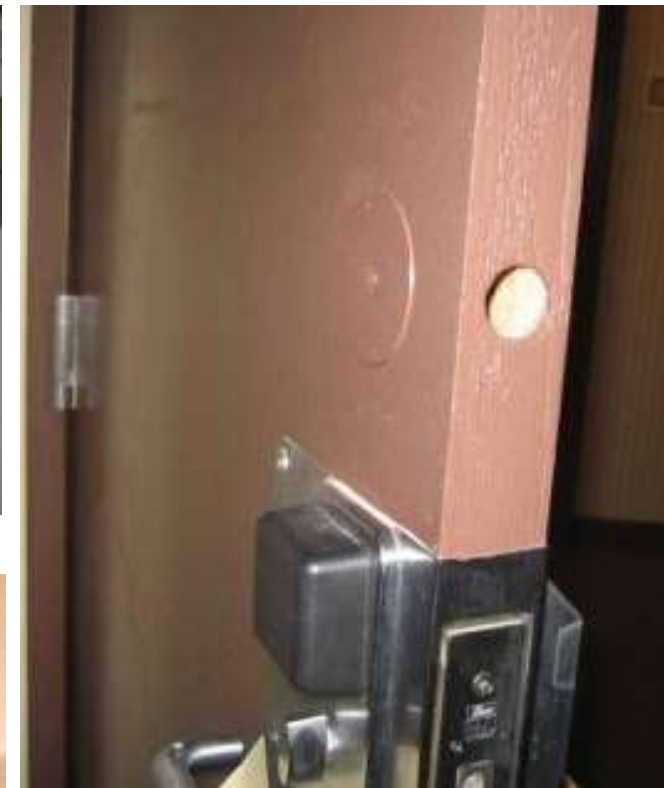
deadbolt never installed on opening
