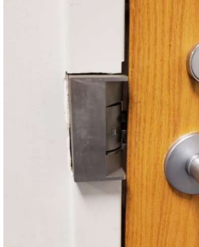
electric strike with mortise lock
