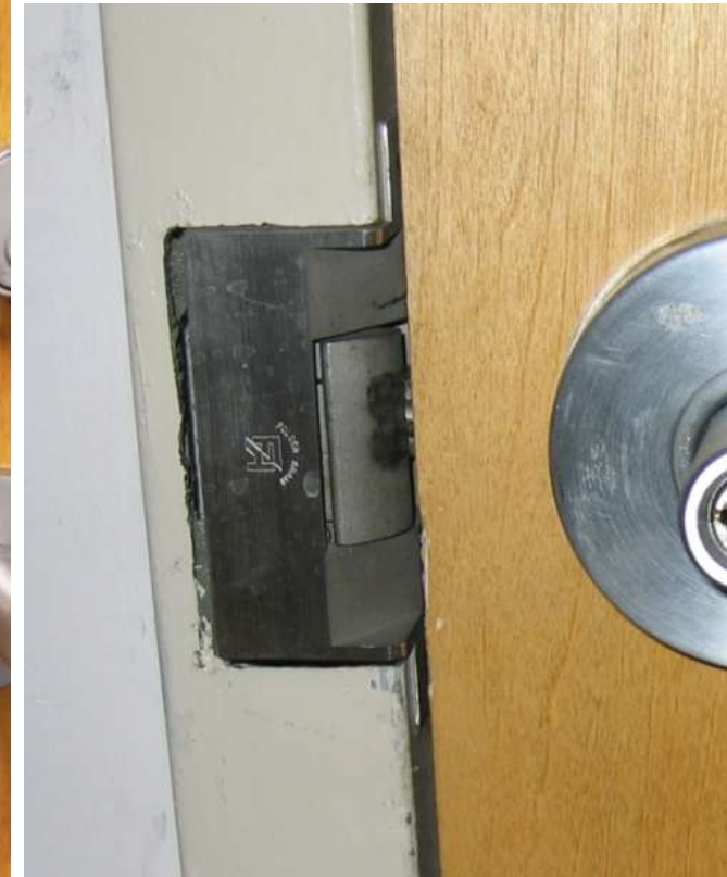
electric strike with cylindrical lock
