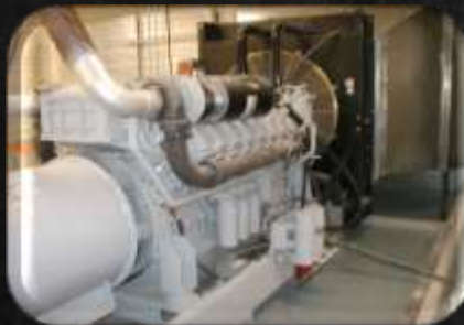
MTU Detroit Diesel
