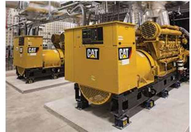
Hospital Back-up Generators
