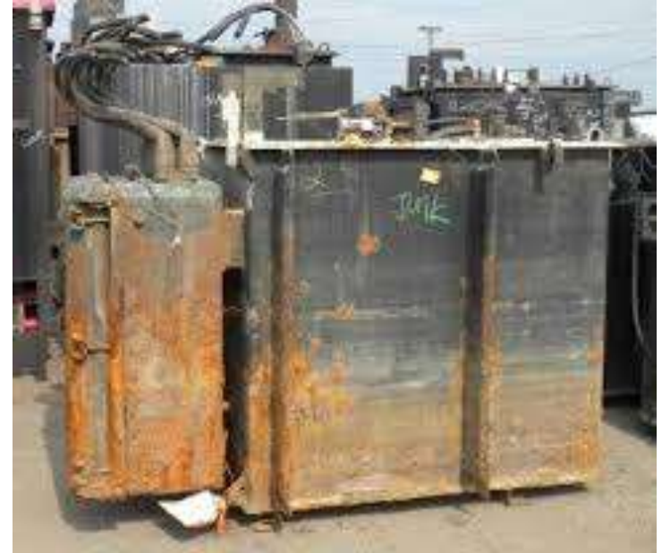
Example of a Aged/Rusted Dry-Type Transformer – ABB.com
