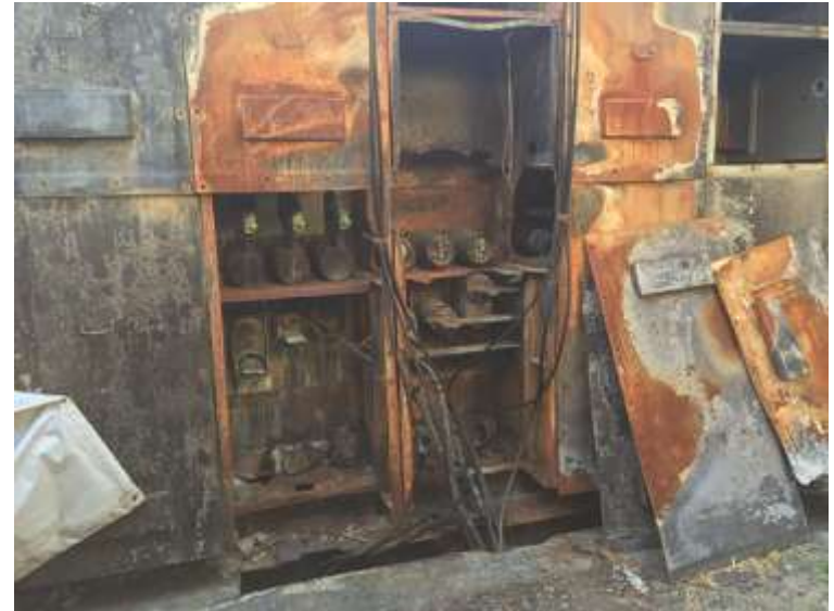
Example of catastrophic failure of Medium Voltage Switchgear
