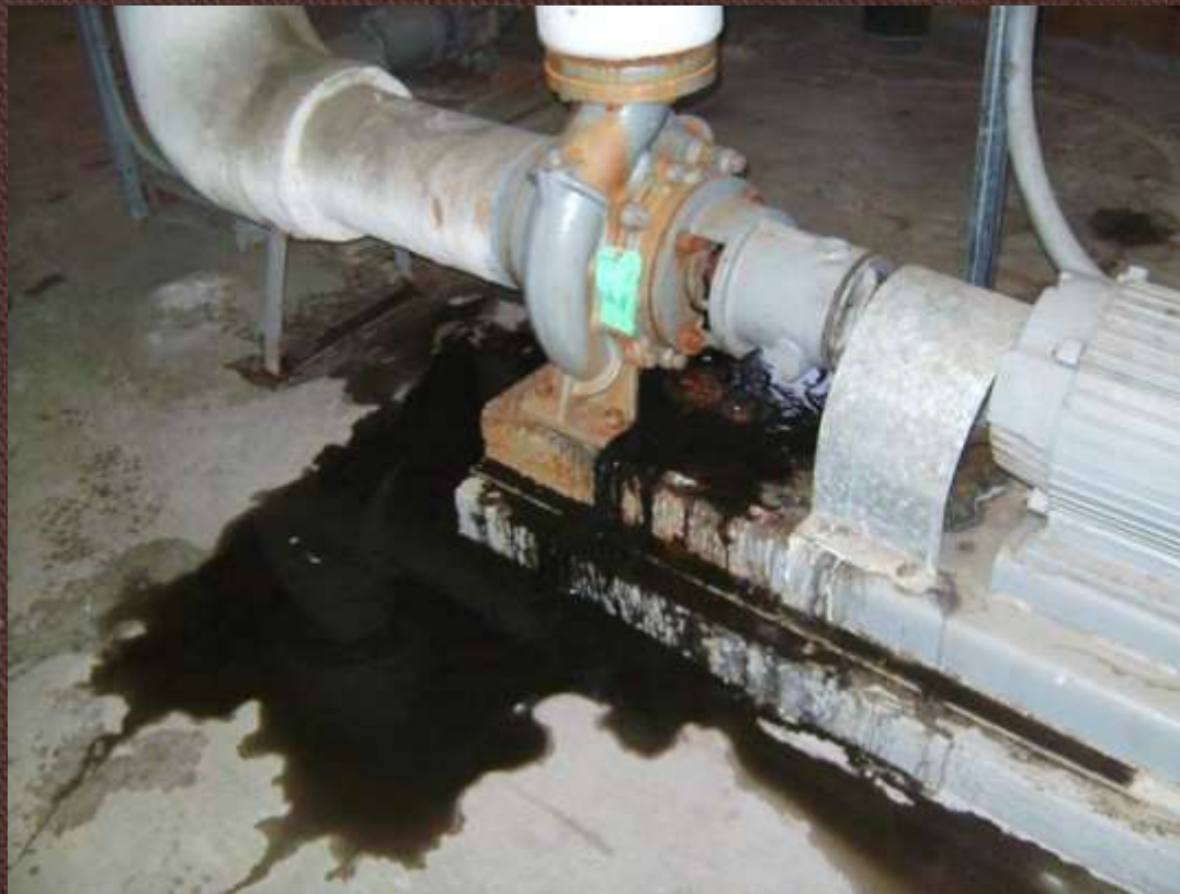
Worn pump seals
